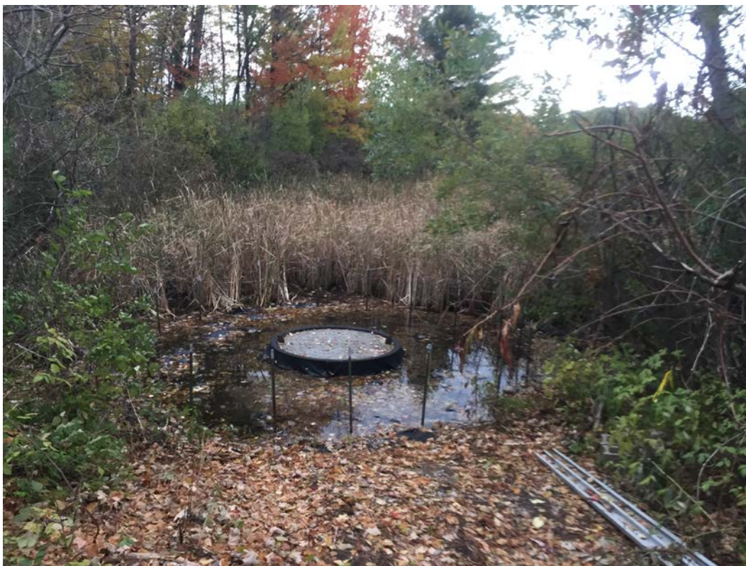
Riser/Intake Structure in Pond Connected to Silver Lake
