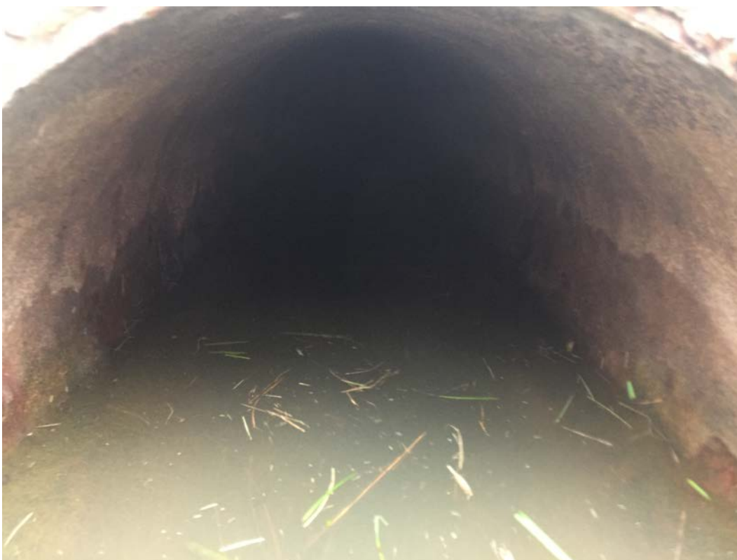
Interior of 14" Diameter Ductile Iron Discharge Pipe
