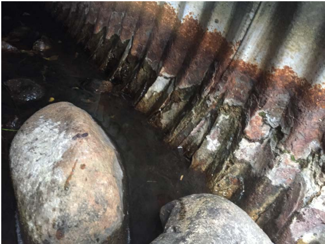
Failing Culvert Downstream of Cox Pond
