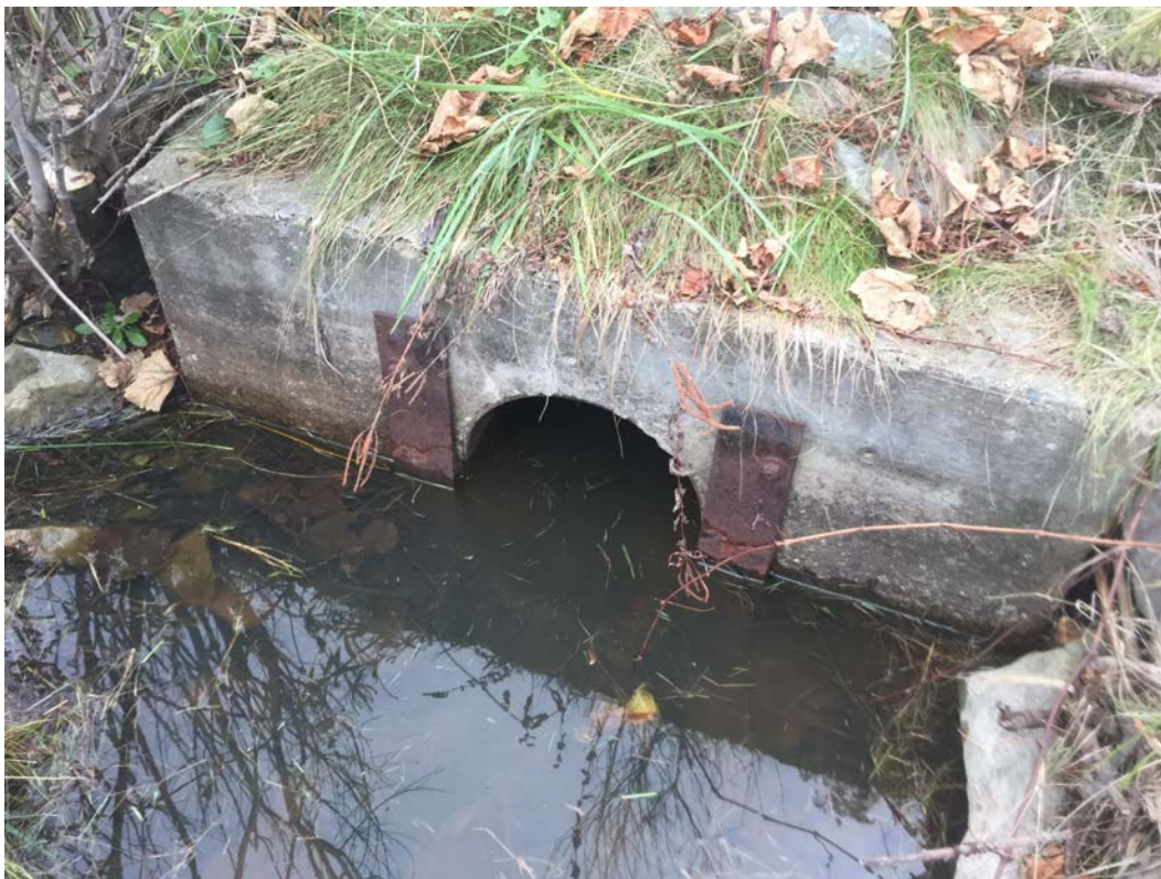
Downstream End of 14" Diameter Discharge Pipe
