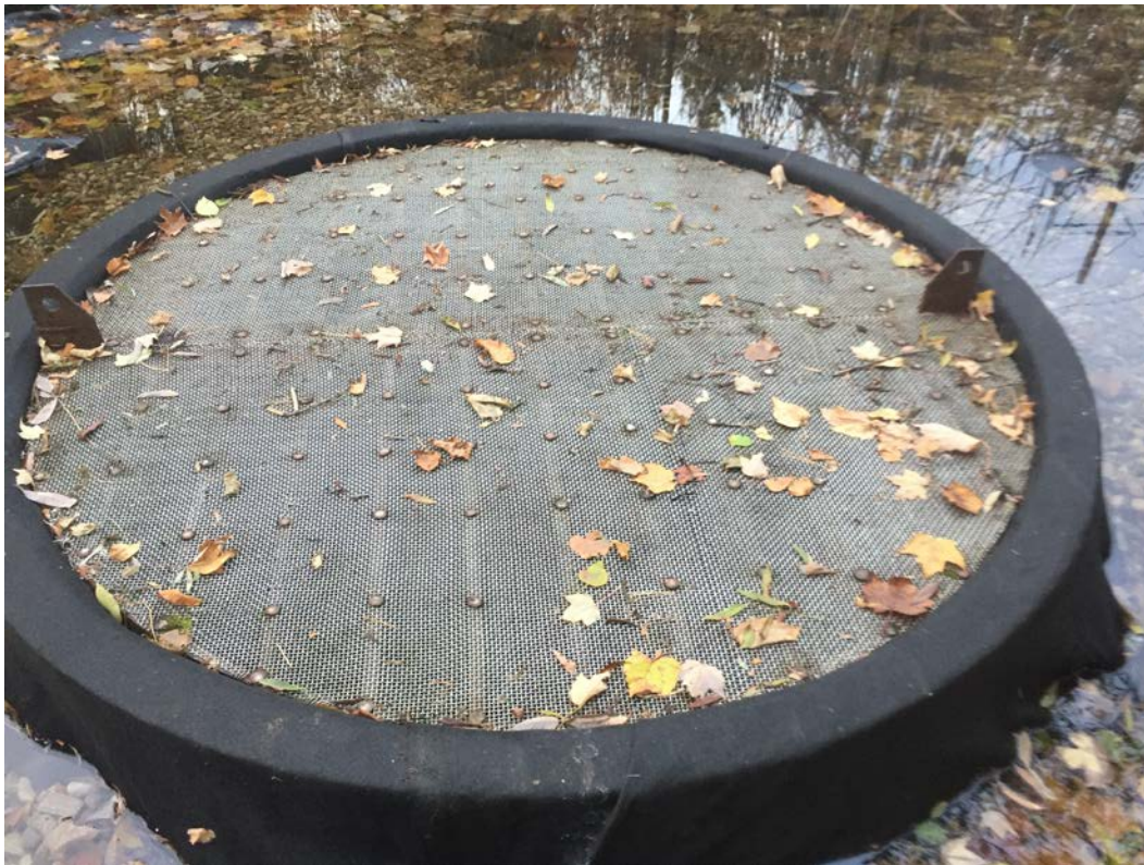
Trash Rack Over Riser/Intake Structure
