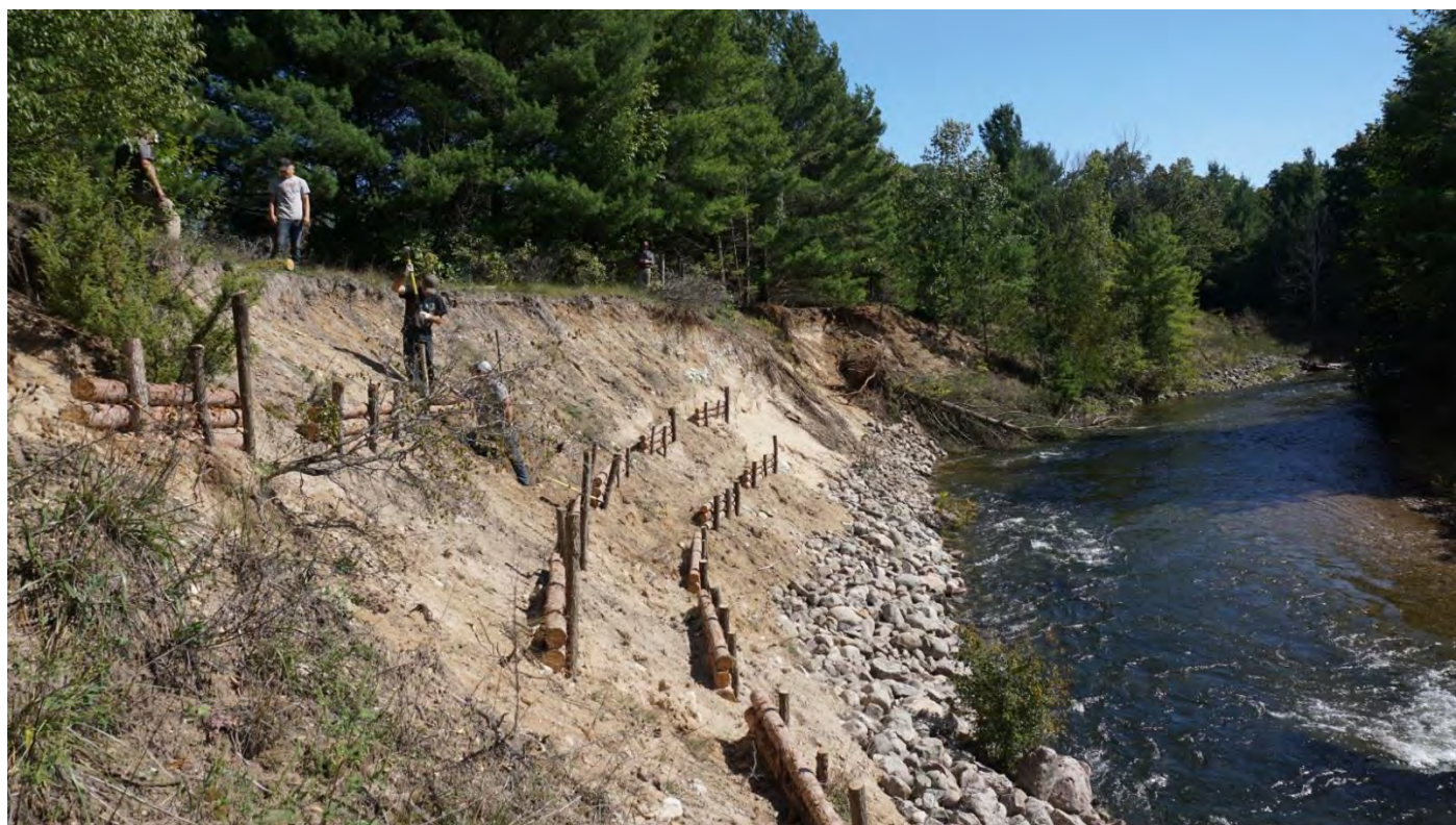
Site #BRD-S117 – Rock placed at the toe & log terracing underway
