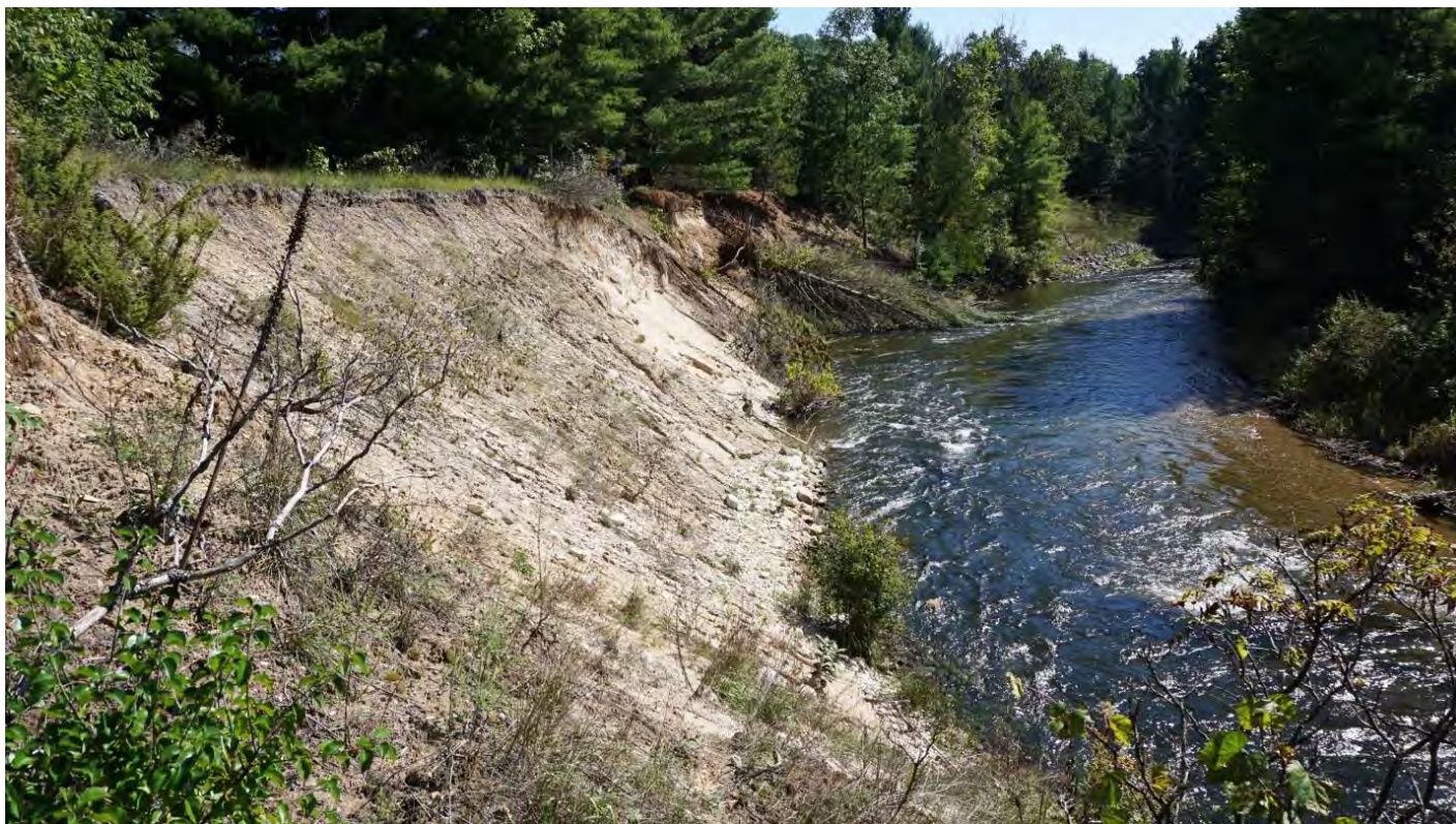
Site #BRD-S117 – Rock placed at the toe & log terracing underway
