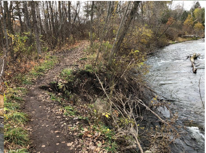
Site #2 – 75' Eroding bank immediately upstream of Site #1. Note how the bank is cutting into the hiking trail. The bank is undercutting and will soon fall into the river.
